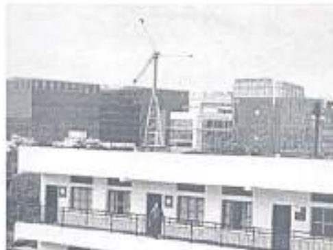
Figure 5-18: Micro wind mill installed in SVP block
