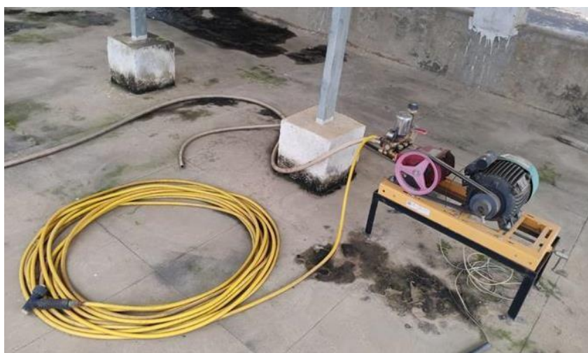
Figure 5-10 Pressurized water cleaning for SRTPV systems
