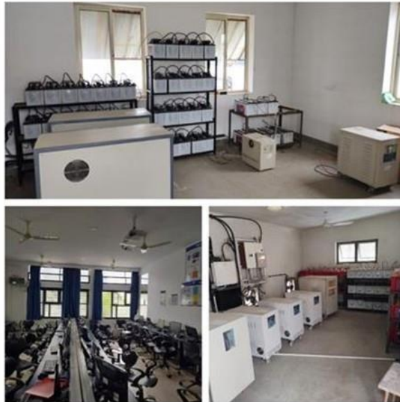
Figure 5-11: Well-ventilated and day-light integrated rooms
