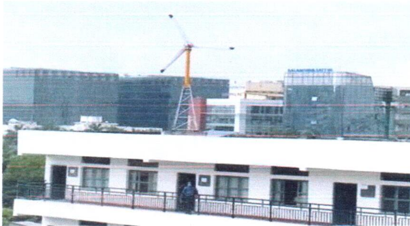
Micro wind mill installed in SVP block
