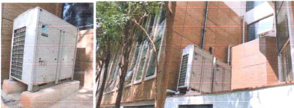
VRV Air Conditioning Unit
